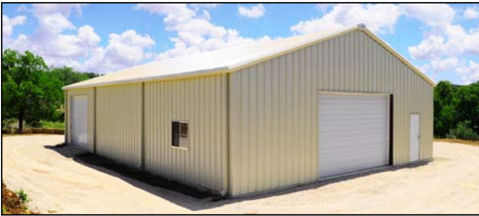
Maintenance Building - Almost Completed
