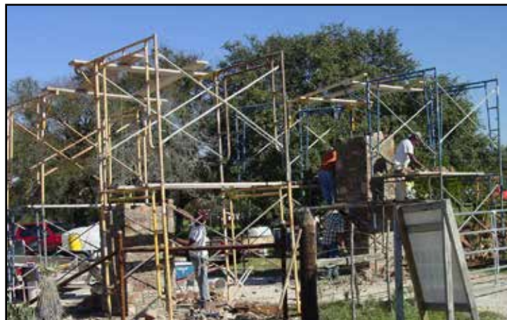
Building the Front Gate
